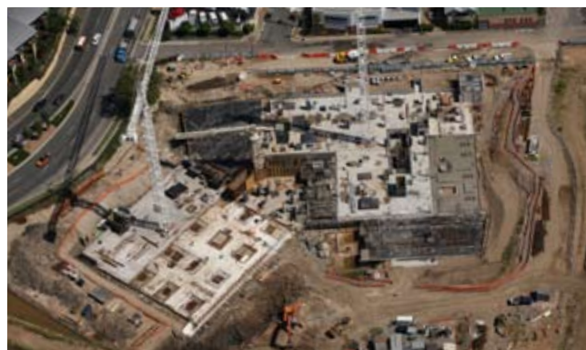
Aerial photograph of Riverpark Building site on 12 February 2009 showing the current status of the works; with two cranes installed and operational, bulk earthworks completed, basement levels substantially completed and works commencing to the ground floor entry level.
