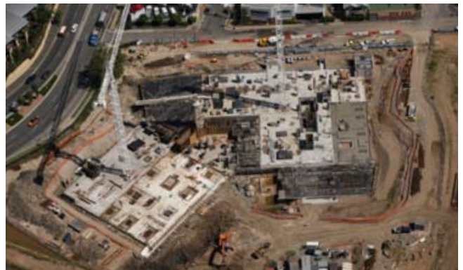
Aerial photograph of Riverpark Building site on 12 February 2009 showing the current status of the works; with two cranes installed and operational, bulk earthworks completed, basement levels substantially completed and works commencing to the ground floor entry level.
